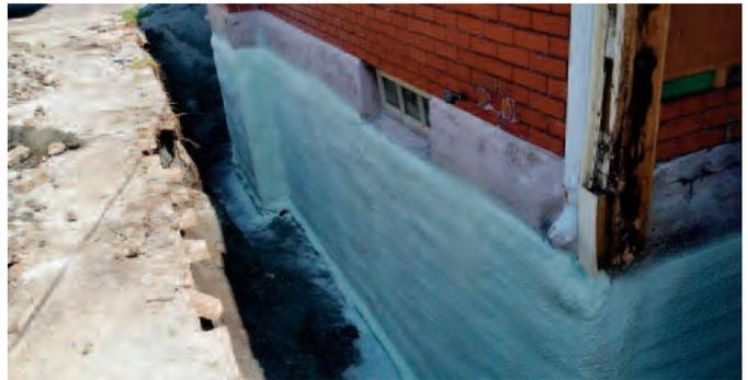
When an old foundation is excavated, it is the ideal time to insulate from the exterior with Heatlok spray foam.
